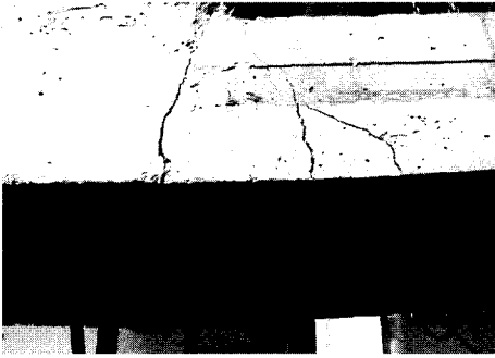
Fig. 19 Initial and final crackings of J-1-S specimen
