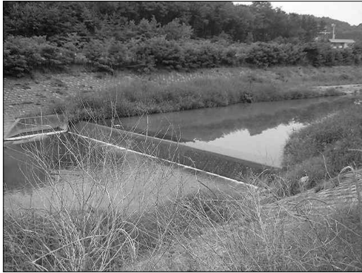
Fig. 13. The flood control structures in Tahndong stream
