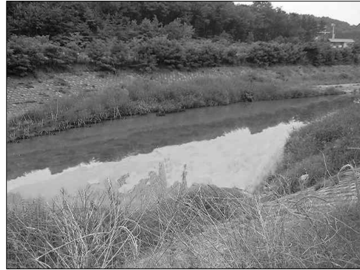
Fig. 14. After Removing the dam
