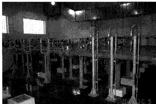
Fig. 5 Reference Turbine Flowmeter Unit
