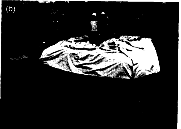
Fig. 7. Lining around the remediation site with impermeable fabric.
