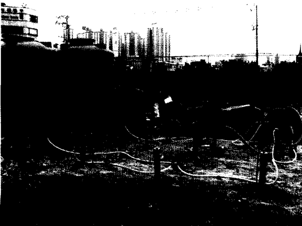
Fig. 8. In-situ soil flushing system in the remediation site.
