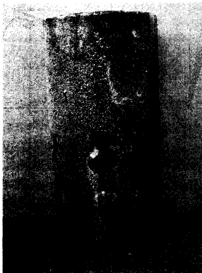
Photo 3 Pop-out of non aging EAFSA concrete (28 days)
