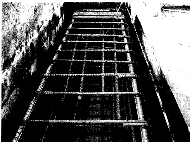
Fig. 4 Reinforcement for specimen RB500
