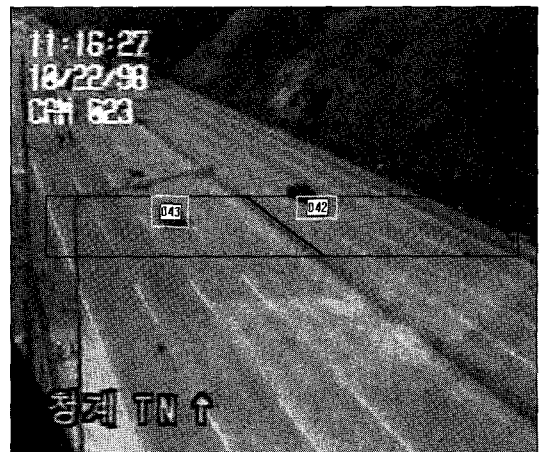
(a) the front of Chungkye Tunnel
