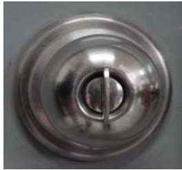
Figure 1. Cylindrical lock(interior).
