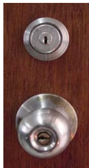
Figure 4. Cylindrical and auxiliary locks mounted on a door(exterior).
