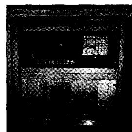
(a) Master controller(upper), DSP controller(lower)
