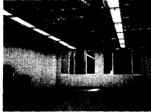
Fig. 18 Inside view of simulator equipped with new HVAC system.
