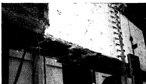
Fig. 12 Specimen RF2-UEB2 at failure (rupture after debonding started at mid-span)
