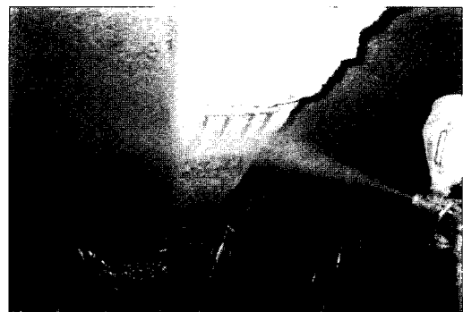
Fig. 8. Photo of applying method of sprinkling with polymer cement material.
