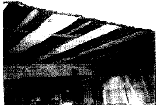
Fig. 7. Photo of applying method of reinforcing with carbon fiber.
