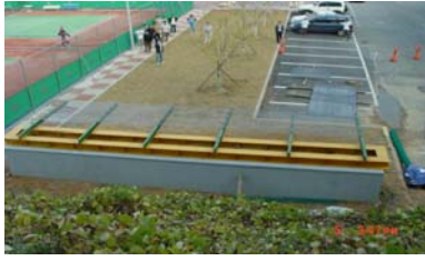
(b) Installation of expanded metal rockfall protection fence
