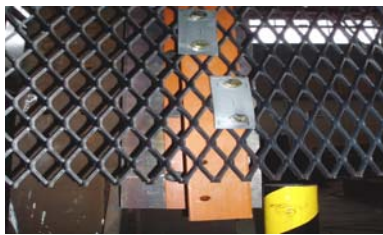
Fig. 5. Connection between support and expanded metal
