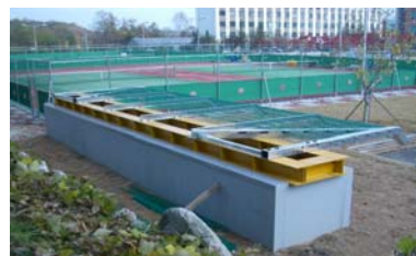
(a) Installation of typical rockfall protection fence
