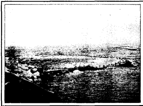
Fig. 3. Photograph of seawater exchange breakwater install
