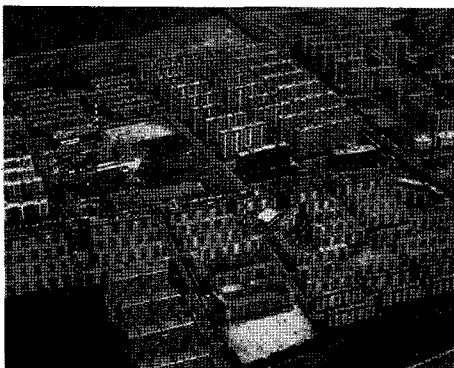
<Figure 3> Apartment complex with uniformed appearance.
