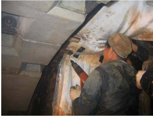
Figure 10. Bullflex Installation
