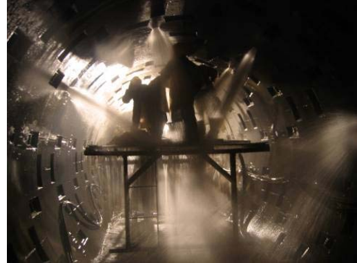
Figure 11. Backfill Grouting
