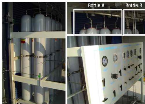
Fig. 2. Propellant/Coolant Pressurization System
