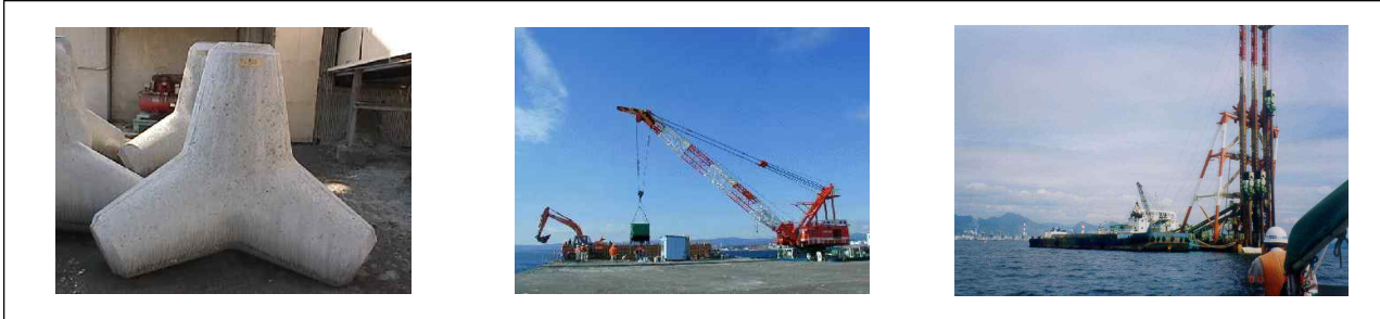
Fig. 2 Use present condition of Japanese copper slag(Tetrapod for seashore, bed plate works of harbor, Sand file works from left)
