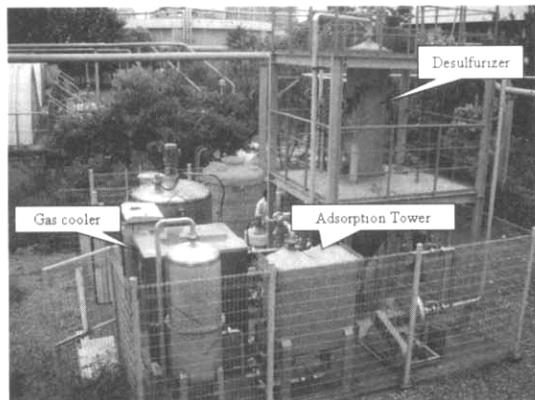
Fig. 8. Photography of Gas Purification Process.
