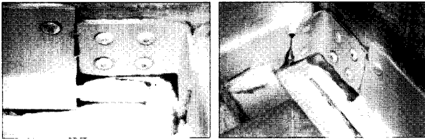
(b) Car end areas of the stainless steel underframe.
