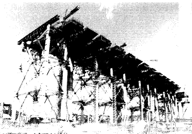
Fig. 10 Back Span Falsework - East Side
