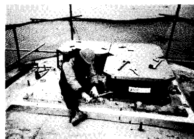
〈Figure 5〉 Kwangan bridge with lead rubber bearing
