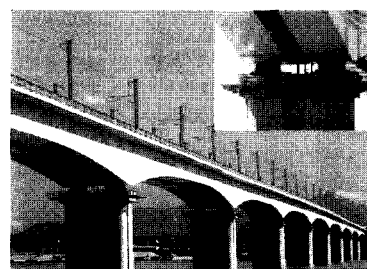
(b) New bridge
