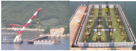
(e) PC house 거치 (f) PC house 세팅 완료
