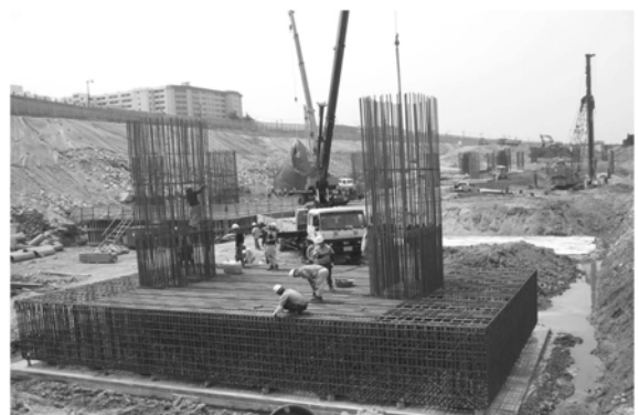
Fig. 2 Foundation concrete of pier
