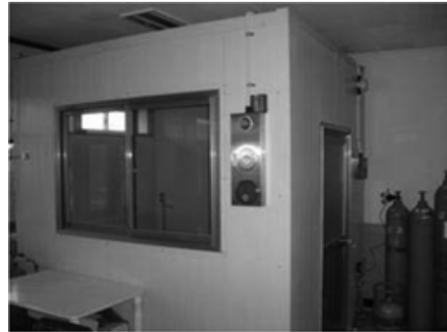
(a) Window (vent 1) and doorway (vent 2)
