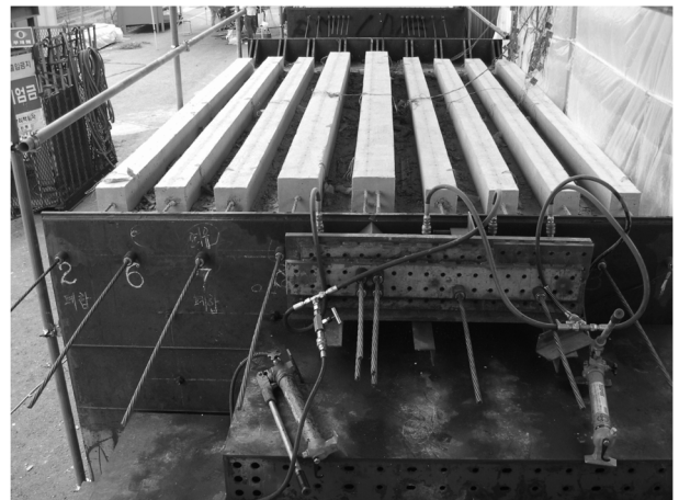
Fig. 4 Testing members and prestressing frame
