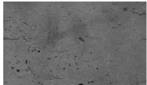
(a) Artificial crack healing section (before)
