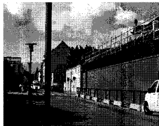
Fig. 5. Simple 3-dimensional temporary fence, Denmark.
