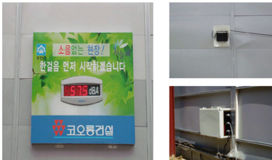
Fig. 1 Whole view of automatic noise measuring system
