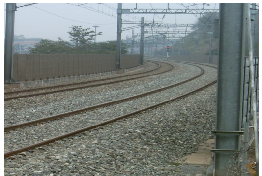
Fig. 4 Steel box bridge and ballast track
