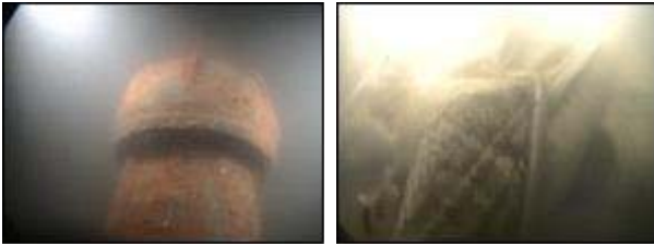
Fig. 5. Cast iron pipe and concrete bag.
