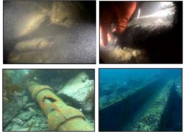
Fig. 6. Damage of HVDC cable.
