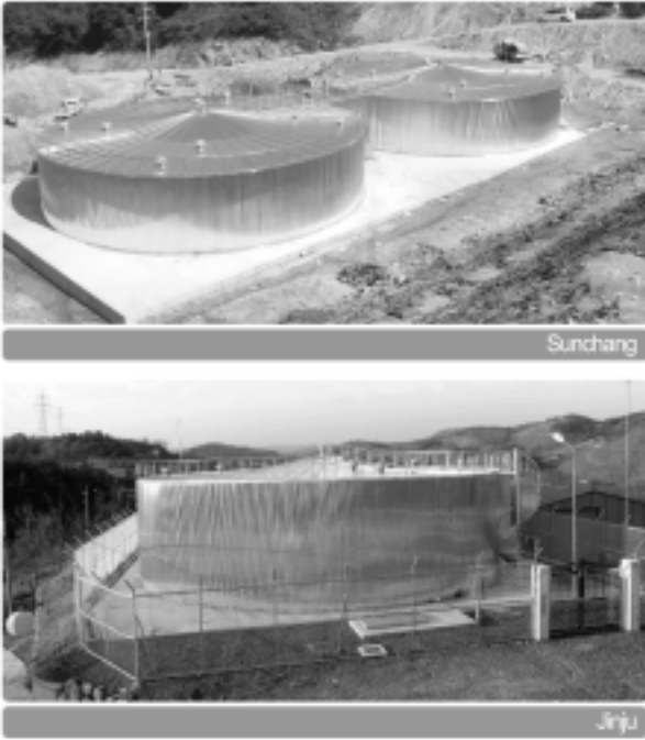
Fig. 1. Circular water tanks.
