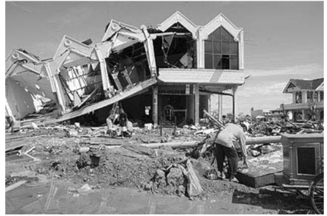
Photo 2. Houses damaged by Indian ocean tsunami (2004)
