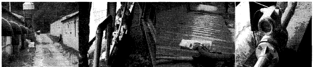
Fig. 1. Flowmeter installed at the pig barn to measure the daily amount of swine slurry.
