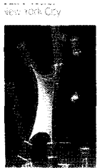
NEW YORK CITY 2008 competition sponsored by the local chapter of the AIA, A&O fabricated a delicate 19-foot-tall structure using 3D printing technology. The freestyle object is made up of uniquely scaled, twisted, and nested hexagons. The architects printed the tower in 15-brush sections and spliced the pieces together with complex but ultimately invisible joints.
