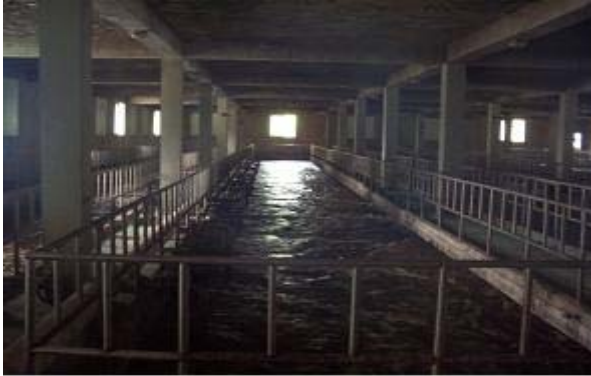
Fig. 2. Scene of B3 reactor
