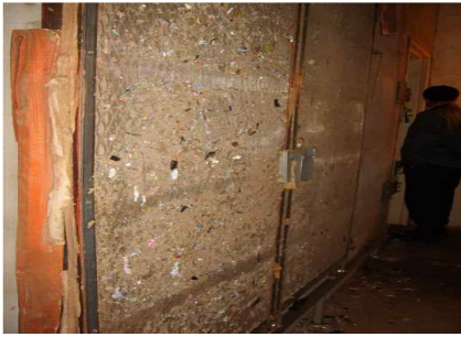
Fig. 5 View of filter room
