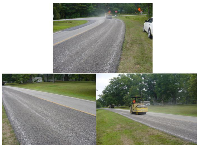
Figure 7. Uneven rolling under steel wheel roller
