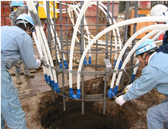
Fig. 3 U-tube installation.
