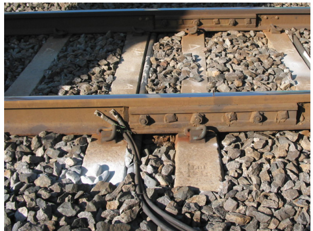
Fig. 7 A joint of rail
