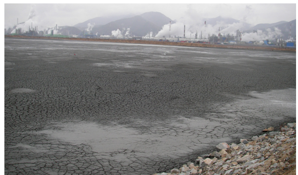
Fig. 2 Soft ground surface when 2~3 years have elapsed since hydraulic fill was finished
