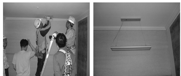
(a) Installing shape at apartment house in daegu (in 2008)
