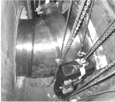
Fig. 5 MSIP application at Salem unit 1
