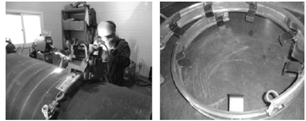
(a) Welding carriage (b) Pipe guide rail
