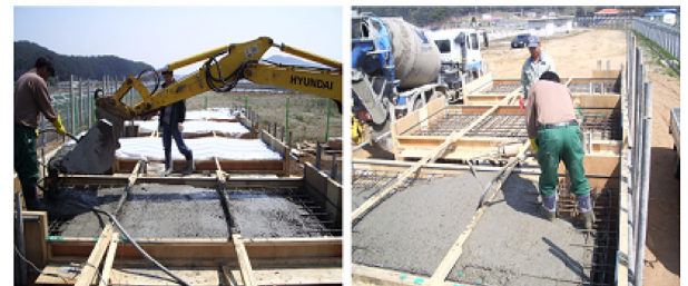
(b) PA concrete placing
