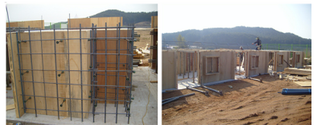
(a) Steel caging and forming
