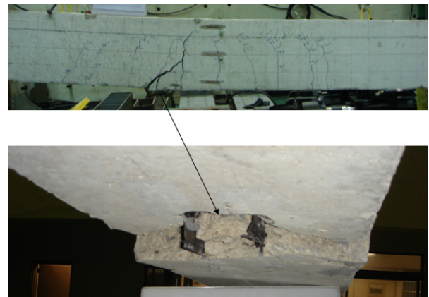
Fig. 3 Failure mode for beam NSM2-32
