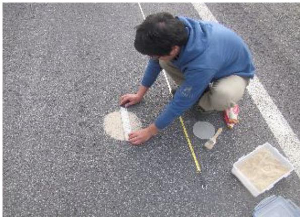
(a) Sand Patch Test on the Asphalt Section
