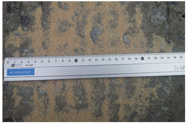
(b) Sand Patch Test on the Concrete Section
