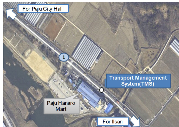
Fig. 1 Location of Transport Management System (TMS) (Hanaro Mart Intersection, Jori-up, Paju, Kyunggi-do)
