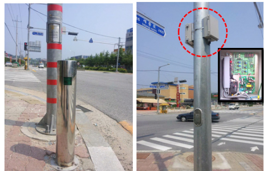
Figure 5. Examples of controller for in-pavement flashing light
