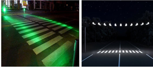
Figure 1. Examples of crosswalks upper-lighting system
