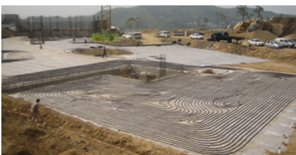
Fig. 3 Photograph of energy-slab installation.
